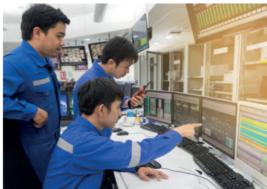
By adding replicas of the Operator Consoles and DCS softcontrollers, digital twins are converted into full Direct-Connect OTSs
